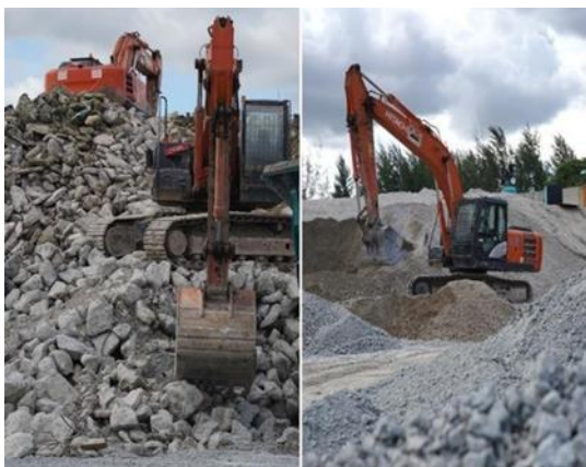
Fig. 1: Collection of demolished concrete
