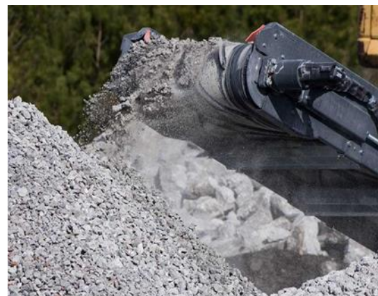
Fig. 2: Recycling of demolished concrete
